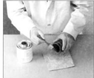
Apply a second full even layer of cement to the pipe. Assemble parts QUICKLY! Parts must be assembled while cement is still fluid. If assembly is interrupted, recoat parts and assemble. Push pipe FULLY into fitting, using a turning motion, if possible, of 1/8 to 1/4 turn, until it bottoms. Hold them together for 15 - 30 seconds to offset tendency of pipe to move out of fittings. With a rag, wipe off excess bead of cement from juncture of pipe and fitting.
