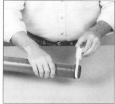
Thread the fitting onto the pipe and hand tighten. Further tighten the fitting (one to two turns past hand tight) by using a strap wrench only.
