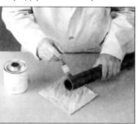
Apply a medium layer of cement to the fitting socket. Do not let the cement puddle. Also, when joining
