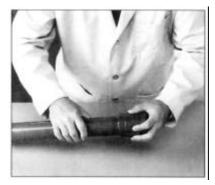
Note: For pipe sizes 6" and larger, two people will be required, a mechanical forcing device should be used, and the joint should be held together for up to 3 minutes.
