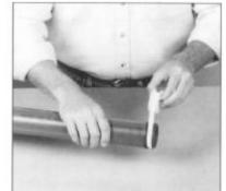
Thread the fitting onto the pipe and hand tighten. Further tighten the fitting (one to two turns past hand tight) by using a
