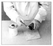
Apply a second full even layer of cement to the pipe. Assemble parts QUICKLY! Parts must be assembled while cement is still fluid. If assembly is interrupted, recoat parts and assemble. Push pipe FULLY into fitting, using a turning motion, if possible,
